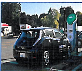
Castle Rock Electric Vehicle Charging Station
